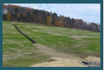
**Temporary slope drains** use flexible tubing or a conduit that extends from the top to the bottom of a cut or fill slope.
