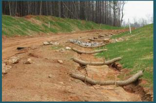
**Check dams** are constructed of rock or other materials across a drainage ditch to mitigate erosion by reducing water flow velocity.
