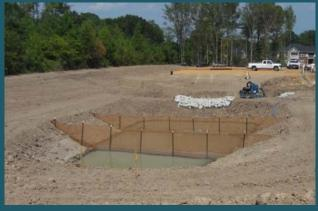
Sediment basins are low earthen dams across drainage ways that create a temporary storage pool.
